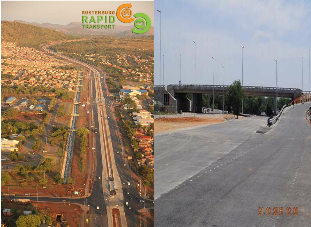
Picture 1: Phase 1A Tlhabane Section (left) and Phase 1B Ramochana Bridge (Right)
